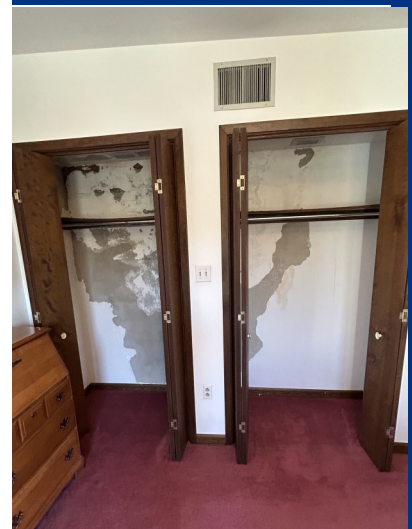
Water Mitigation at CTK
