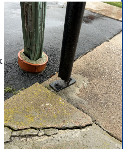
Railing Replacement at IC
